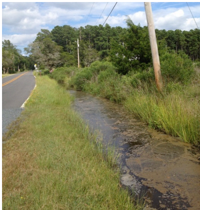
Photo: Tidal ditches in Oriole that often overflow onto roadways, representing one of many concerns voiced at our December meetings (see below for more details).
